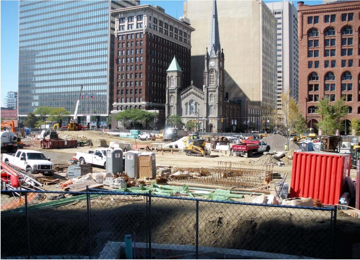
During Construction! Wait until next June.
